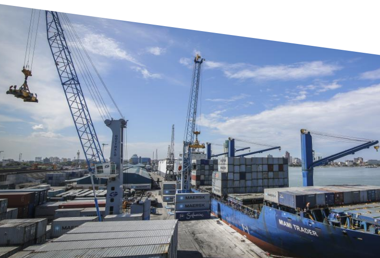
Hafen von Dar es Salaam, Tansania, © MLC Properties AG
